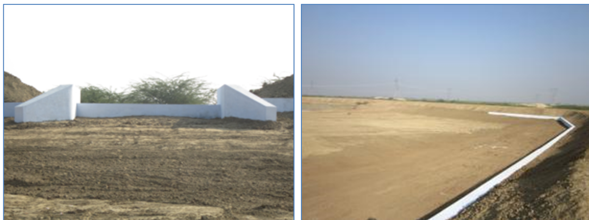
Overflow and Face-wall structure of the pond
